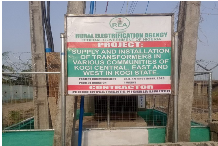
i Installation of Transformers, Okene Kogi State
