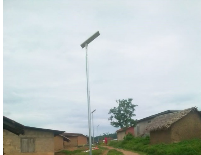
i Solar-powered Streetlights powering a community in Iko Ekperem, Rivers State
