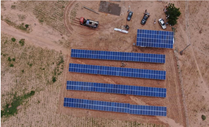
100kWp mini-grid, Eka Awoke Community, Ebonyi State
