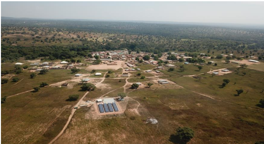
Ariel view of the 64kWp mini-grid, powering Rokota community, Niger State
