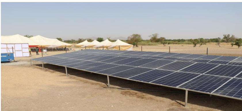
30KwP mini-grid at Mbela Lagaje community, Adamawa State
