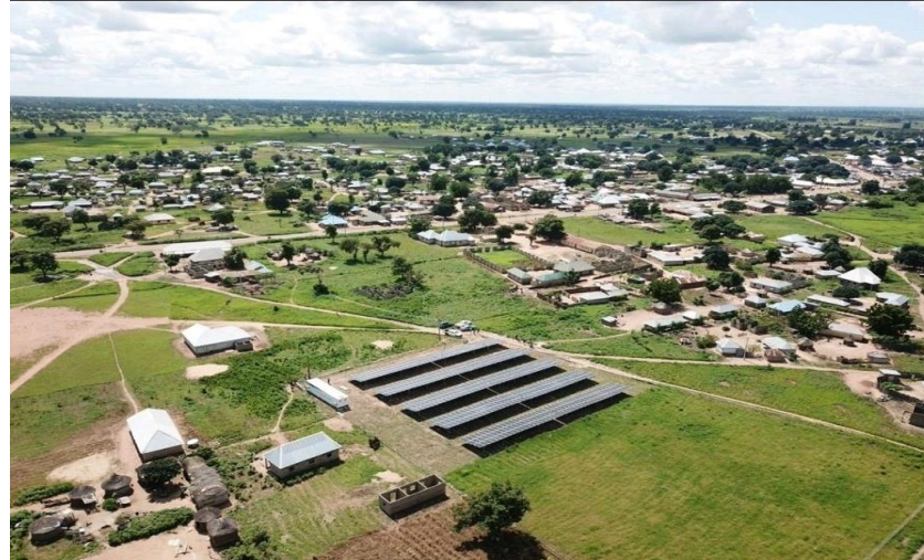
234kWp mini-grid, Shimankar, Niger State
