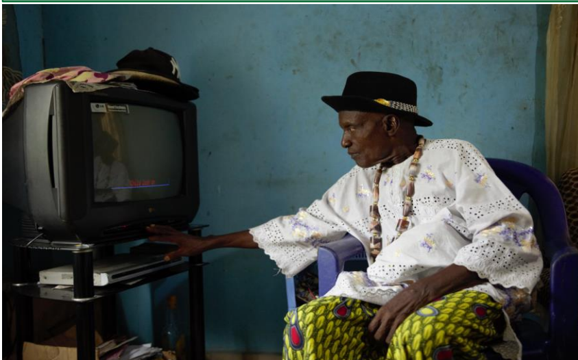
The village chief catching up with the news, powered by the 100KW mini grid, Akpabom, Akwa Ibom
