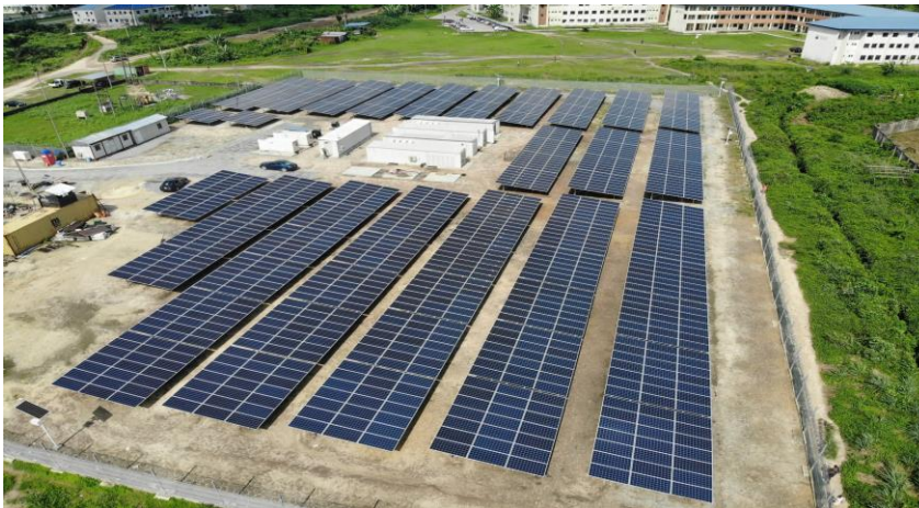
1.35MW Solar Hybrid Project at the Federal University of Petroleum, Effurun (FUPRE), Delta State
