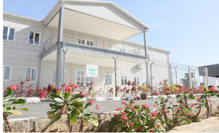
EEP WTC (Workshop and Training Centre), ATBU, Bauchi
