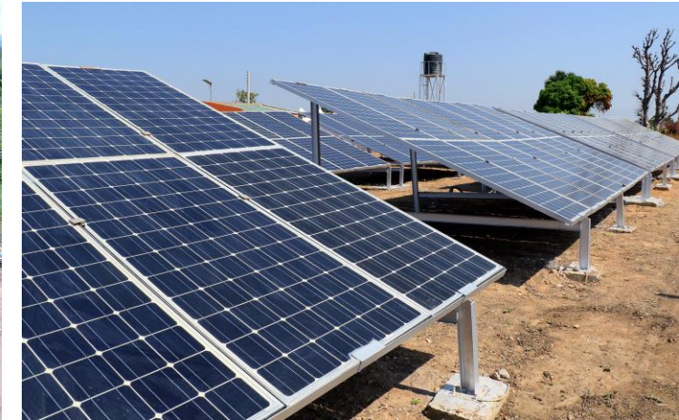
40 kWp mini-grid, Goton Sarki, Niger State
