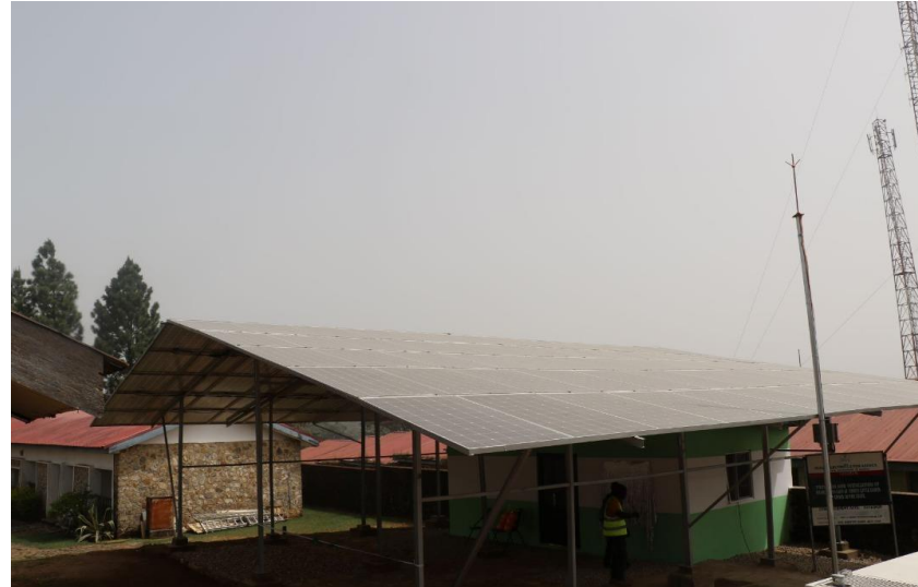
60KwP mini-grid at the Obubudu Cattle Ranch, Cross River State
