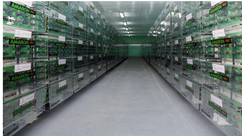
Battery room powering the 8.2MW solar hybrid project in Federal University of Agriculture Markurdi (FUAM)
