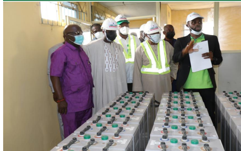
A tour of the battery room of the 100kWp mini-grid, Adebayo community, Edo State
