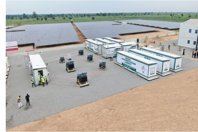
7.1 MW solar hybrid power plant, BUK, Kano
